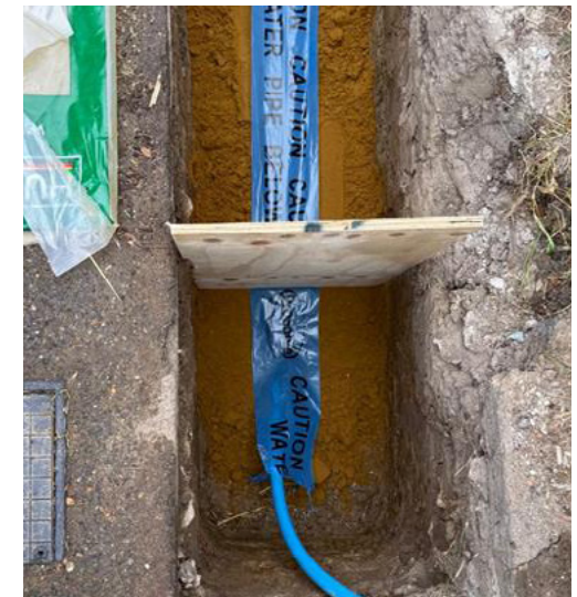
Pipe bedded down with sand
