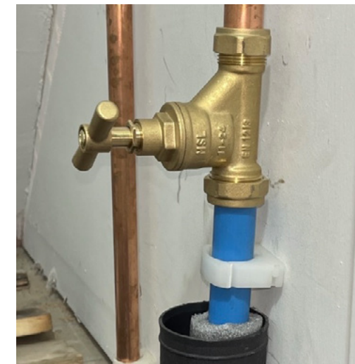
Stop tap (to be installed on both domestic and fire supply)
