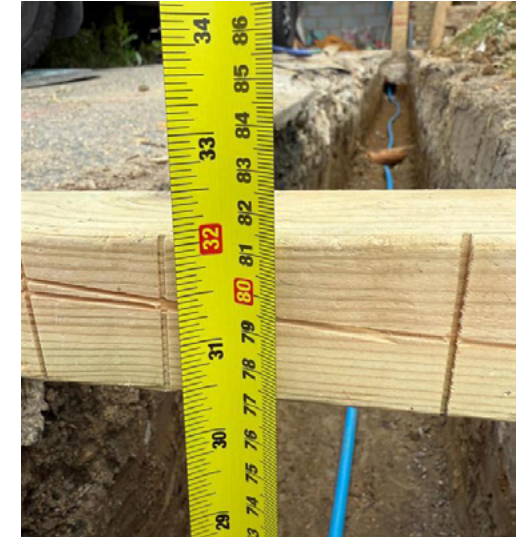
Pipe laid to at least minimum depth
