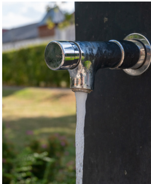
Self-closing, non-concussive tap with no hose union facility
